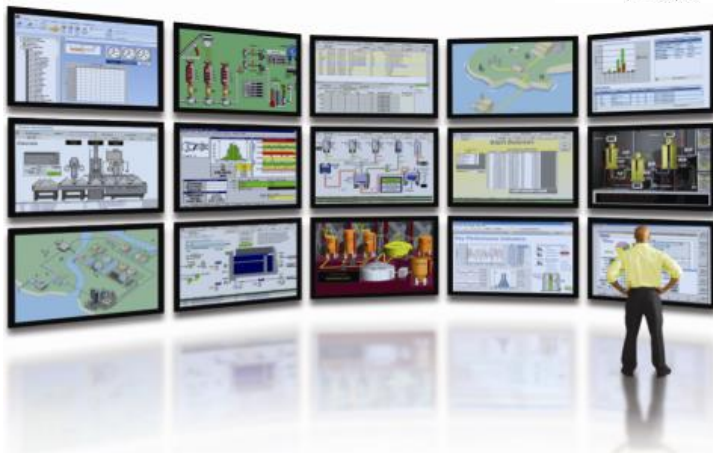
KenerSys Energy Management System
